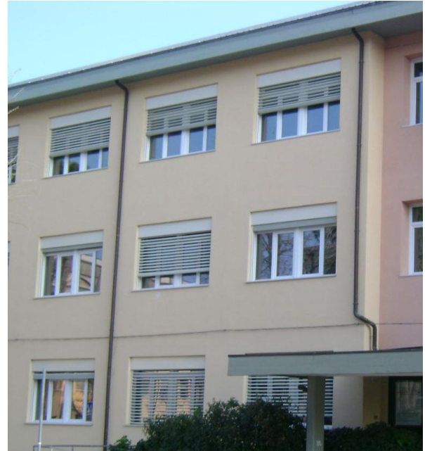
Figure 1: The wooden slats on the left figure can be tilted but not retracted. The shading system defines the façade of the building; on the right figure, fully moveable shading systems are integrated at the window level and can be operated by the users according to their requirements [1].
